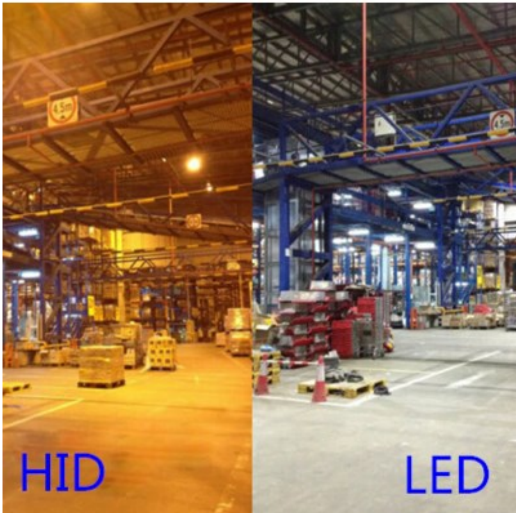
Figure 2: HID lighting systems are prone to “yellowing” after prolonged use while LED systems retain their clarity over time.
