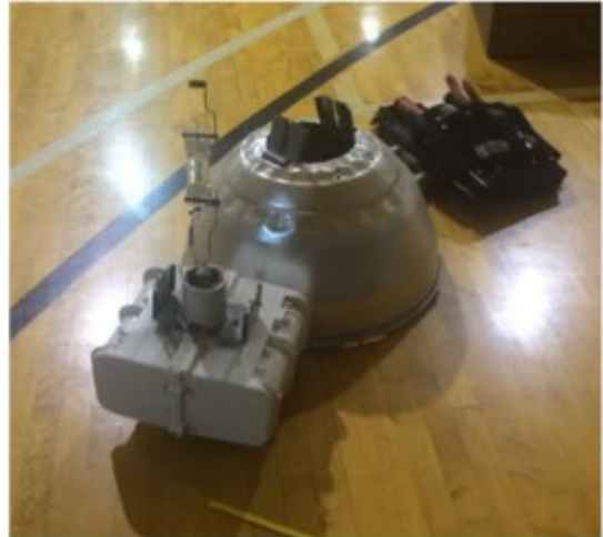
Figure 3: The current HID lights in Walzel Gym.
